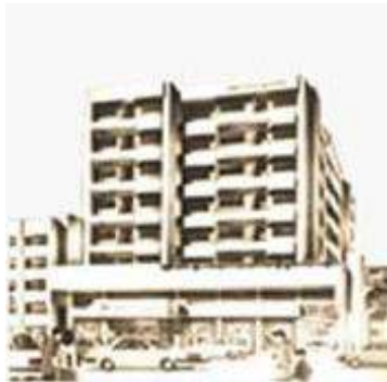
SOLER TOWER RESIDENTIAL, MANILA
