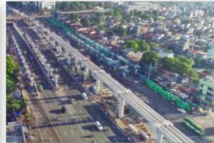
METRO MANILA RAIL TRANSIT SYSTEM LINE 7 (MRT-7)
